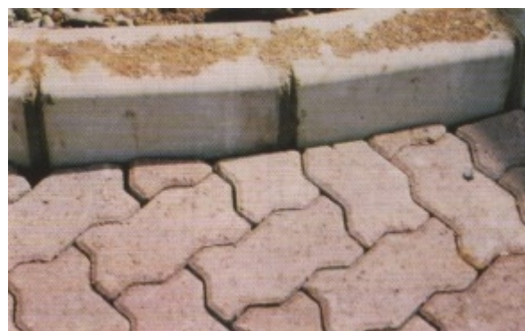
Cutting blocks at edge restraints
