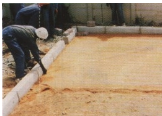
Edge restraints installed before laying commences
