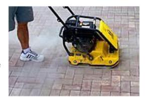
damage to the surface of the pavers. The plate compactor may also move product out of line. New paving must be cordoned off for 7 days, with no pedestrian or vehicle traffic.
