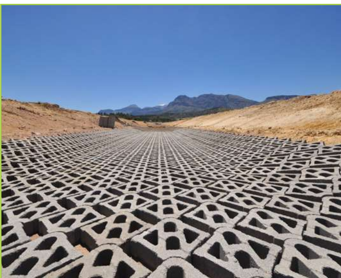
STORM WATER CONTROL & ATTENUATION
