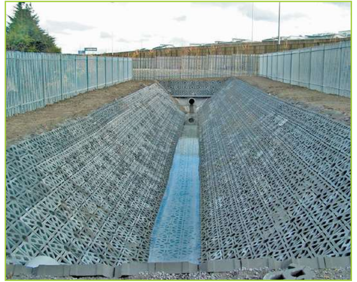
STORM WATER ATTENUATION
