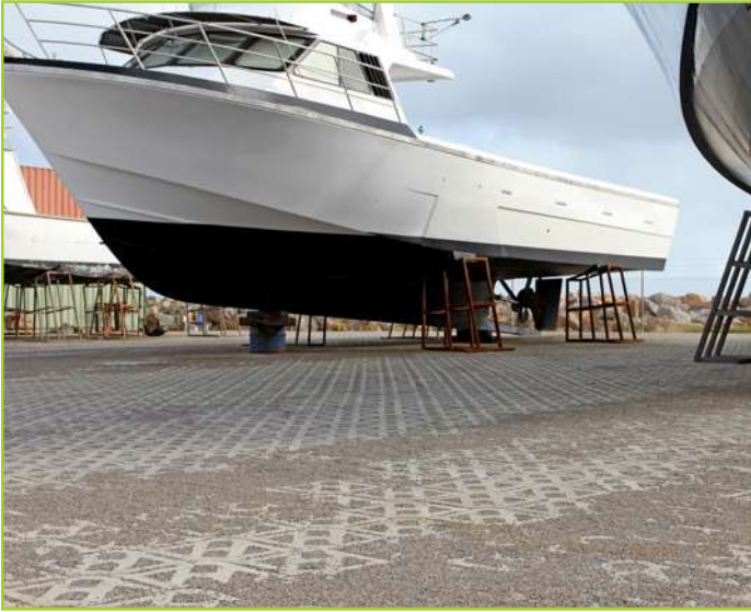
PERMEABLE PAVING FOR 300 TON BOAT LIFTER OPERATION
