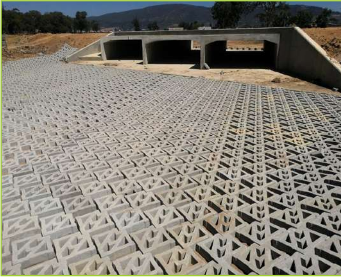
STORM WATER CONTROL AT BRIDGE
