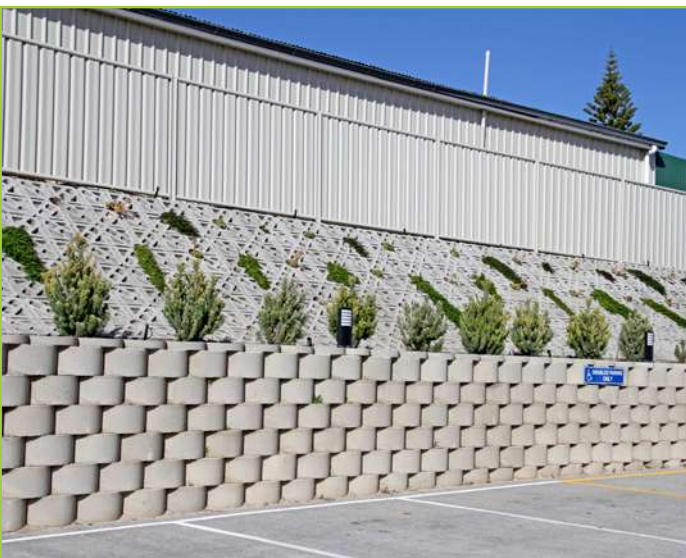
TERRACRETE EROSION CONTROL
