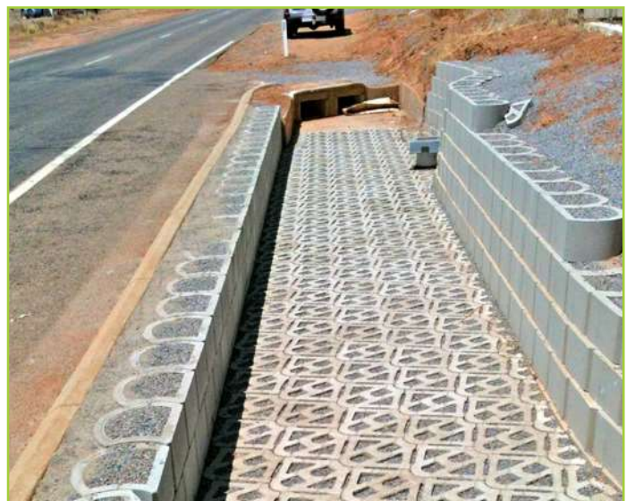
STORM WATER CHANNEL
