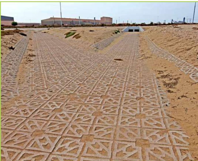
PLANTABLE STORM WATER CONTROL
