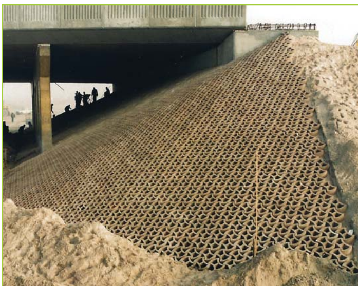
BRIDGE ABUTMENT STABILISATION
