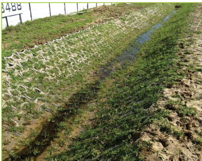
HEAVY EROSION CONTROL FOR A STREAM
