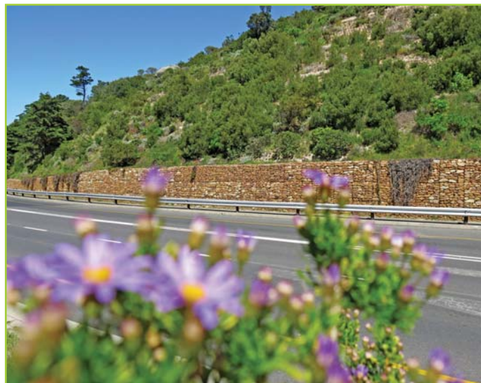
THE SAME INSTALLATION NEXT TO A BUSY ROAD
