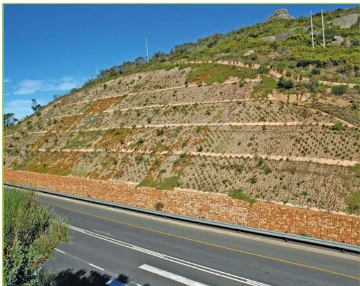
REHAB OF BADLY ERODED AND UNSTABLE CUT SLOPE
