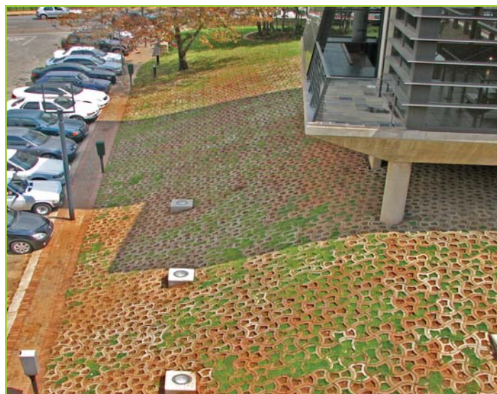
SLOPE STABILISATION AROUND A NEW BUILDING
