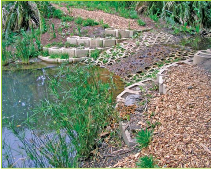
STORM WATER INLET AND WETLAND REHABILITATION
