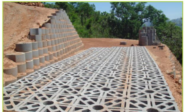
1. **Description:** Permeable Paving Block with two triangular and two arrow shaped openings as shown
