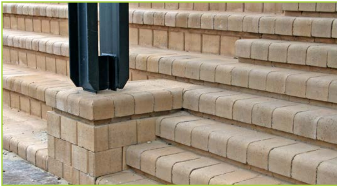
CLOSE UP OF BLOCKS CUT TO SHAPE
