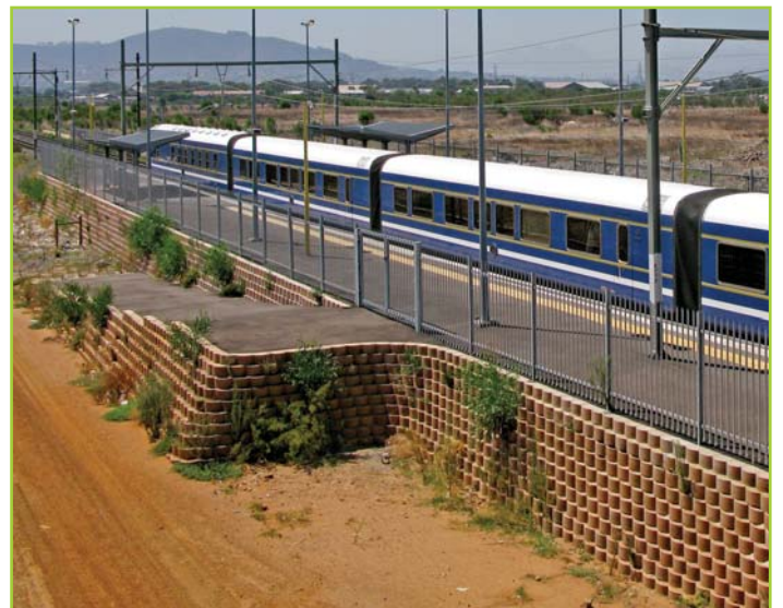
SUPPORTING INFRASTRUCTURE DEVELOPMENT
