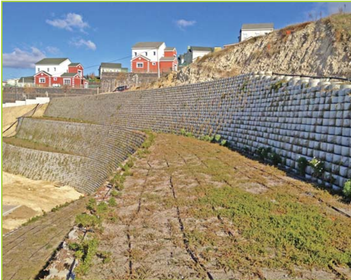
TERRACED RETAINING, HOUSING DEVELOPMENT
