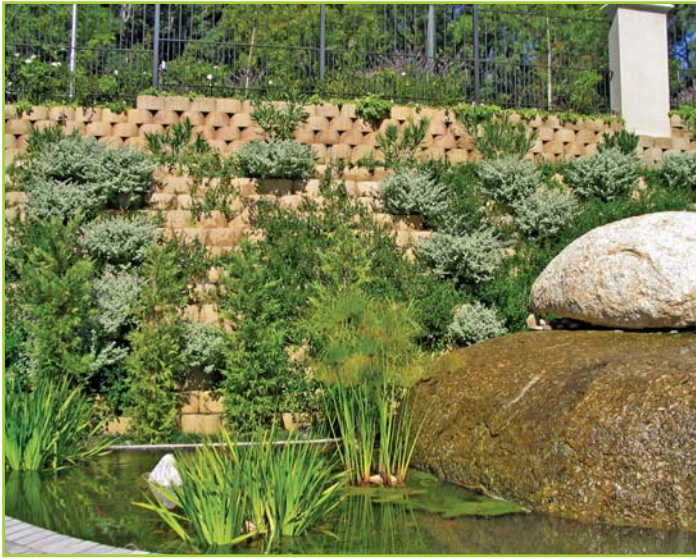
STABILISING AND LANDSCAPING OF CUT & FILL SLOPES
