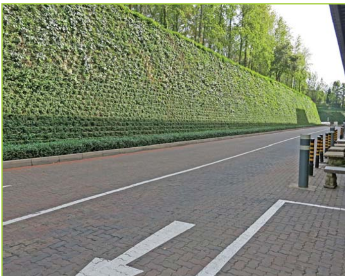
ROADSIDE RETAINING WALL WITH FULL PLANT COVER
