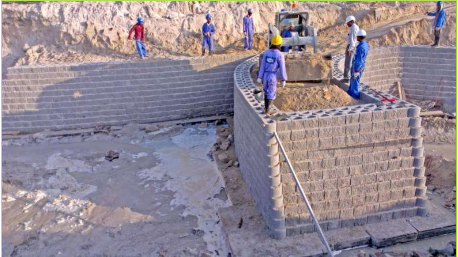
One of the pedestrian ramps under construction
