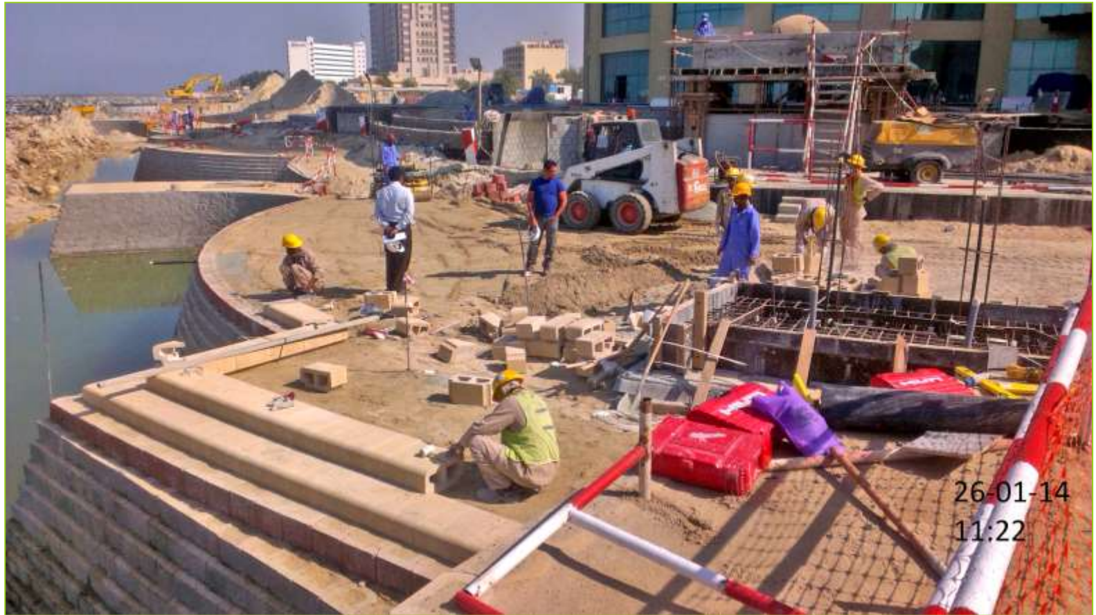
Steps in the process of installation above the drainage layer
